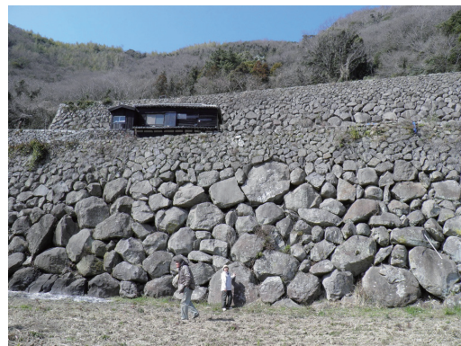
Fig. 18 Nine-meter high stone walls in the paddy field of Iwaishima Island © Hideto KUNIHURO
