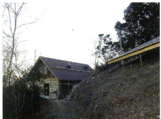
Fig. 15 Hitobito no Tsudoi no Ie (left) and its solar battery panels (right).
